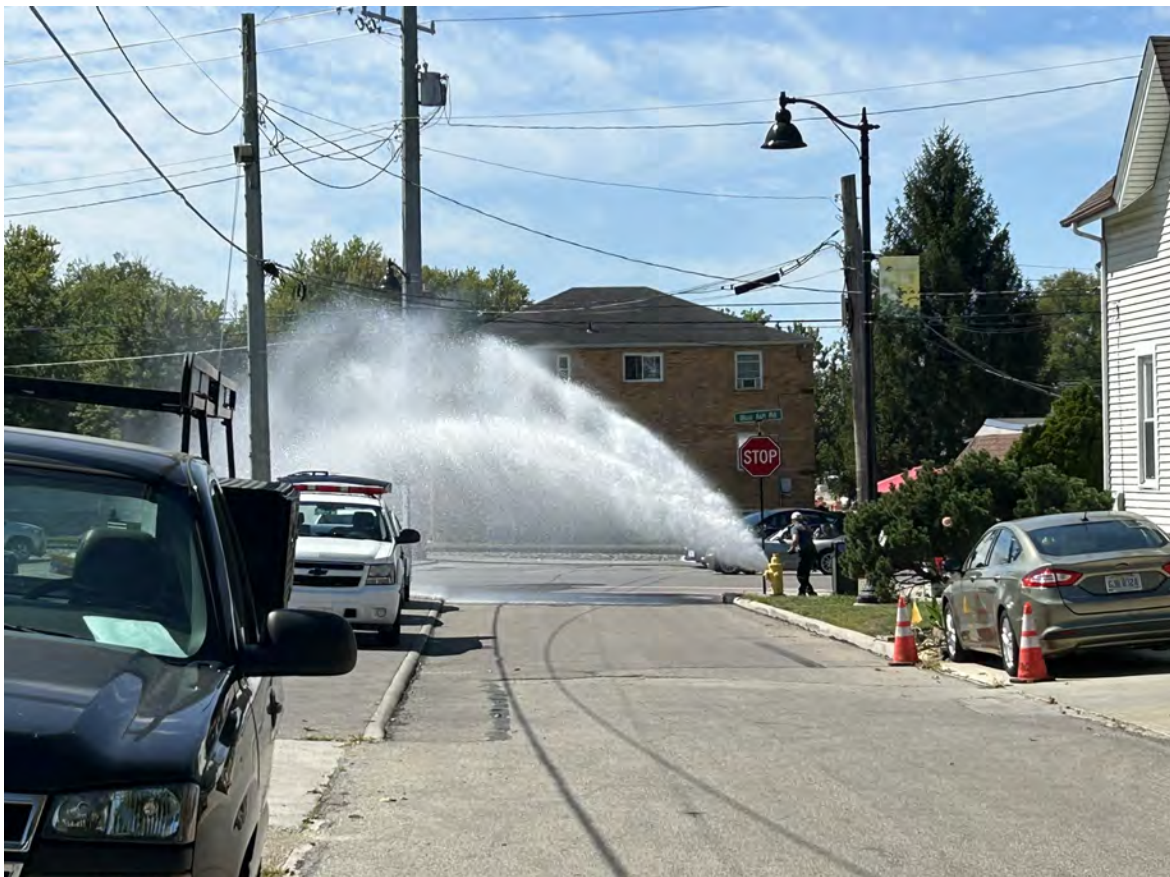
As part of our ISO evaluation, select hydrants throughout the fire district were flowed to calculate the volume of water available for fire suppression. This hydrant, at the intersection of Blue Ash Road and Oakwood Avenue, can deliver up to 1,060 gallons of water per minute.
